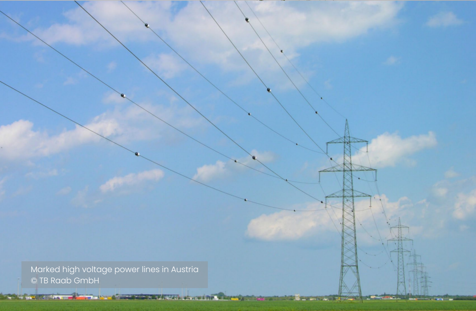
Marking of high voltage power lines in Austria © TB Raab GmbH
